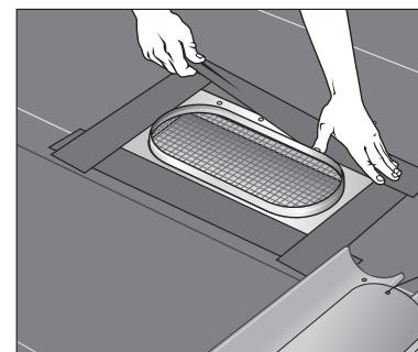
**2. SEAL, ATTACH & FLASH** as shown in Steps 2-4 of the 1-Piece installation instructions. Apply field tile up to the primary vent, nailing tile wire into place.
