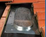
Installed O'Hagin's WEATHERMASTER™ secondary vent cover and primary vent (subflashing) with portions exposed to show rain and snow-resistant interior stainless-steel matrix.
