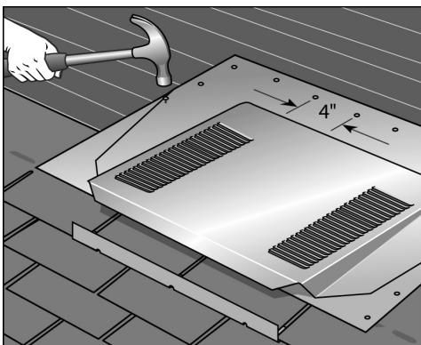
**4. SECURE** at 4-inch centers using roofing nails of sufficient length to penetrate sheathing. **SEAL** all penetrations using locally-approved sealant (Class A where required by code for flame resistance).
