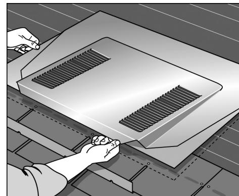
**3. PLACE** vent directly over 11-inch x 11-inch hole using previously marked outline as a guide.
