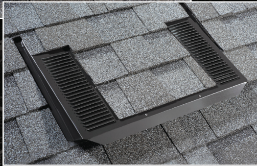
Shingle Over Finish Applied by Installer
