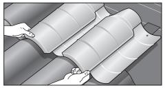
REMOVE surrounding roof tiles, existing secondary vent (cover) and any debris on or near the primary vent (subflashing).
