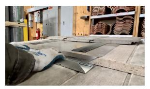
3. Shim below diverter and apply locally approved Class A sealant/adhesive to seal any gaps between flat tiles and diverter.
