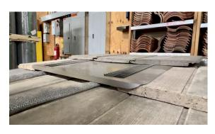
2. Gently apply downward pressure on the 1/8" wire mesh until it slides under the tapered edge of the existing Low Profile "FLAT" tile vent; then continue to slide WUI retro kit until it sits flush with the lower flange of the existing vent.
