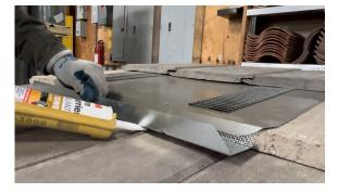
**Note:** The wire mesh rails are flush against the interior of the weather diverters all the way to the back of the Low Profile "FLAT" tile vent.
