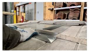
3. Apply locally approved Class A sealant/adhesive to seal any gaps between flat tiles and diverter.
