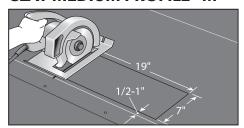
1. MARK & CUT primary vent (sub flashing) opening as shown. Align the bottom of the opening 1/2 to 1 inch above the pan tile layout line as shown. (NOTE: Set blade to the thickness of the sheathing.)
