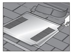
**6. TRIM** roofing material back 1 inch on top and sides of vent cover to allow for proper drainage.
