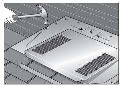
4. SECURE at 4 inch centers, using locally-approved roofing nails or screws of sufficient length to penetrate sheathing. SEAL all penetrations using locally-approved sealant (Class A where required by code for flame and ember resistance).
