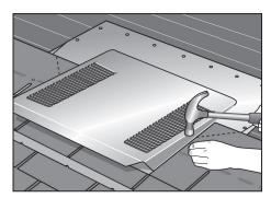
5. COVER with roofing material around vent. Based on local best practices, a 45 degree angle cut must be made on the material terminating at the vent. (See Step 5A if installing shingle-over finish method.
