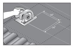
**2. Cut** the 14 x 14 inch hole in the roof deck. (Note: Set blade to the thickness of the sheathing.)
