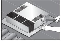
**4. SECURE** vent at 4 inch centers, using locally-approved roofing nails or screws of sufficient length to penetrate sheathing.
