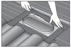
4. FLASH (See No. 1 in the General Instruction Notes below.) When using peel and stick or membrane and mastic methods, apply bottom strip first, then sides, and finally, the top strip.
