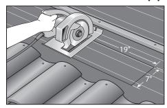
MARK & CUT a 19 inch x 7 inch hole in the roof deck, centered between layout lines and aligned approximately as shown on the exposure lines. (Note: Set blade to the thickness of the sheathing.)
