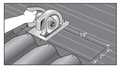
MARK & CUT a 19 inch x 7 inch hole in the roof deck, centered between layout lines and aligned approximately as shown on the exposure lines.
